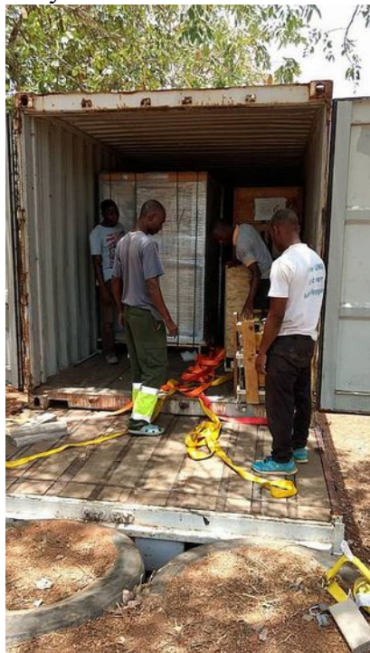
◀ Unloading the transmitter after its arrival.
