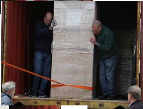
◀ Each transmitter was tilted, then blocked, to allow the forklift to get under the transmitter.
