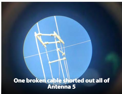
One broken cable shorted out all of Antenna 5
