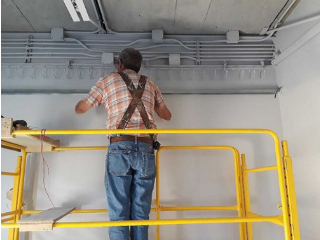
Larry installs one of about 30 light fixtures. At least one wall of each office has reflective lighting using tiny LEDs on self-adhesive tape (~10 LEDs per inch) hidden inside a U-channel, which bathes the wall in light.
