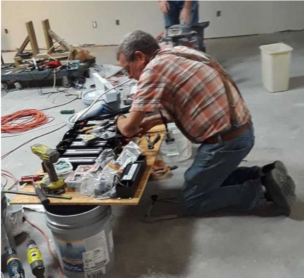
Larry makes a panel by mounting seven 24-volt LED power supplies to power 14 LED light fixtures.
