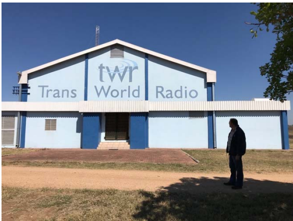
This is a photo of TWR's transmission site in Eswatini.
